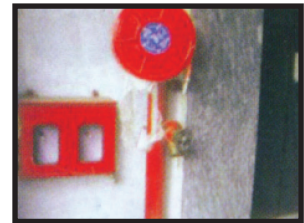
Hose box, Hose reel drums & fittings
